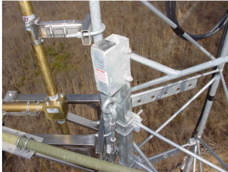
PHOTO SHOWS SAFETY CLIMB AT TOP OF TOWER.
